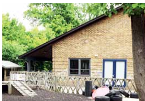
Good: abundant sun heat but with external shading devices, e.g. canopy (top), overhangs (bottom)
